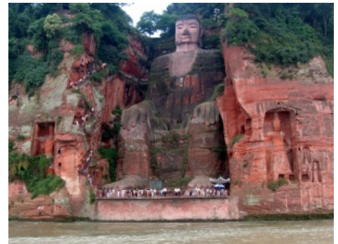
Leshan Buddha in China, 2005, sandstone blackened and corroding from acid rain. Photo by Ariel Steiner (Wikimedia)
