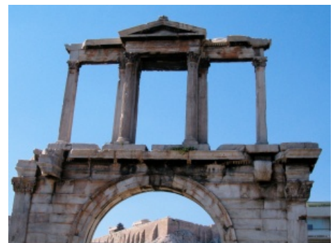
Hadrian's Arch at the Acropolis, Athens, 2005, marble blackened and corroding from acid rain. Photo by Marcok (Wikimedia)
